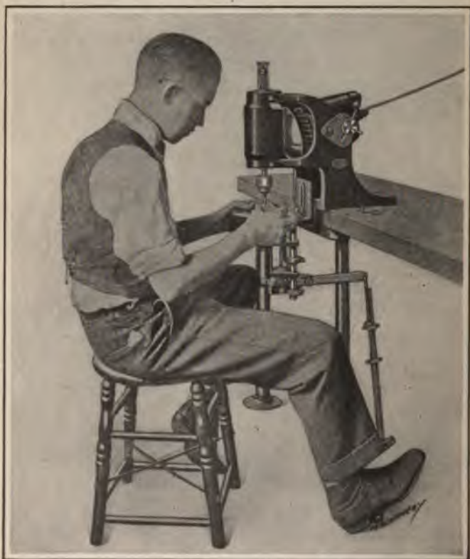
Fig. 7. Anderson Vertical-spindle Tapping Machine
